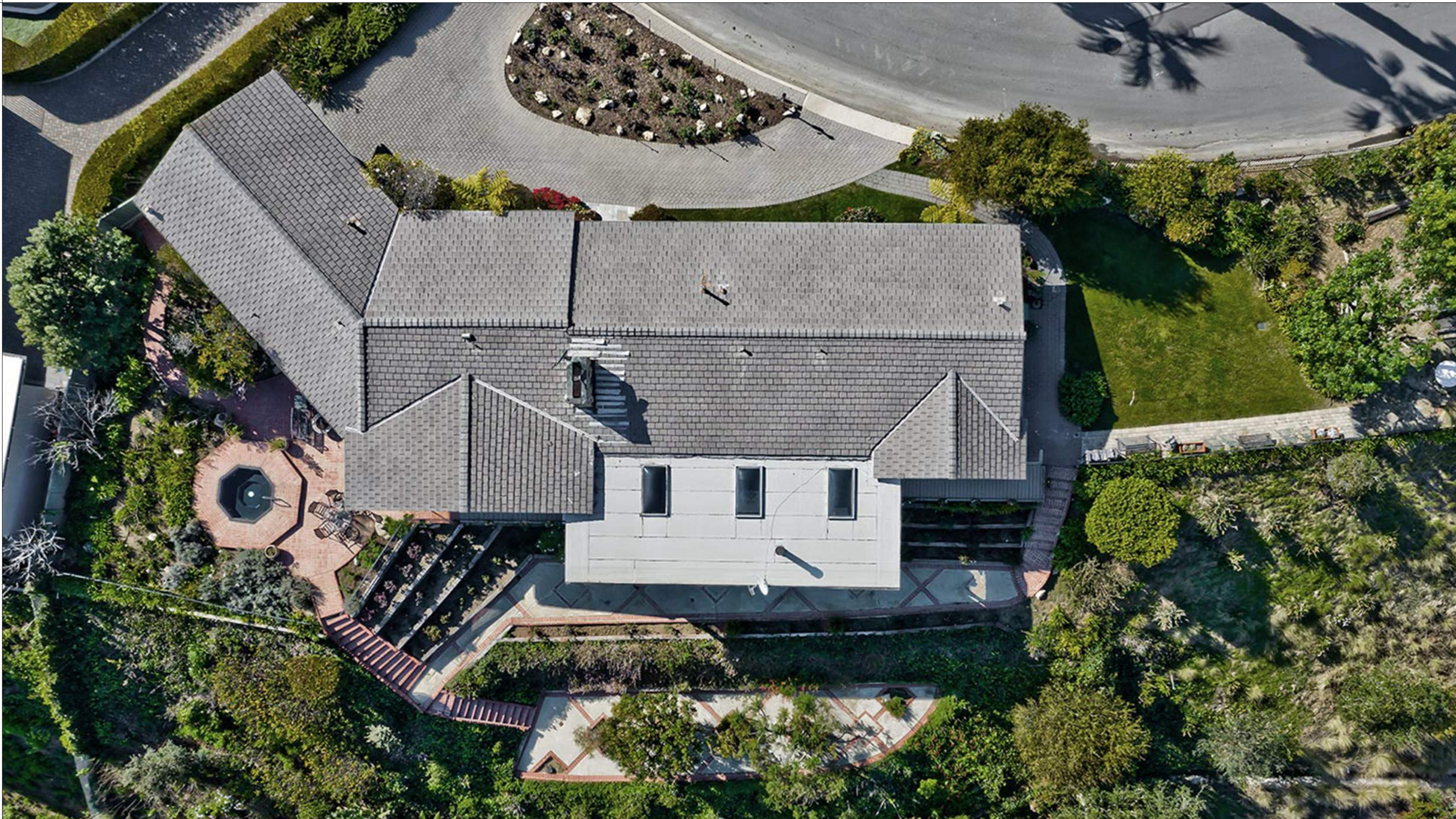
6 ROOF VIEW (E)
