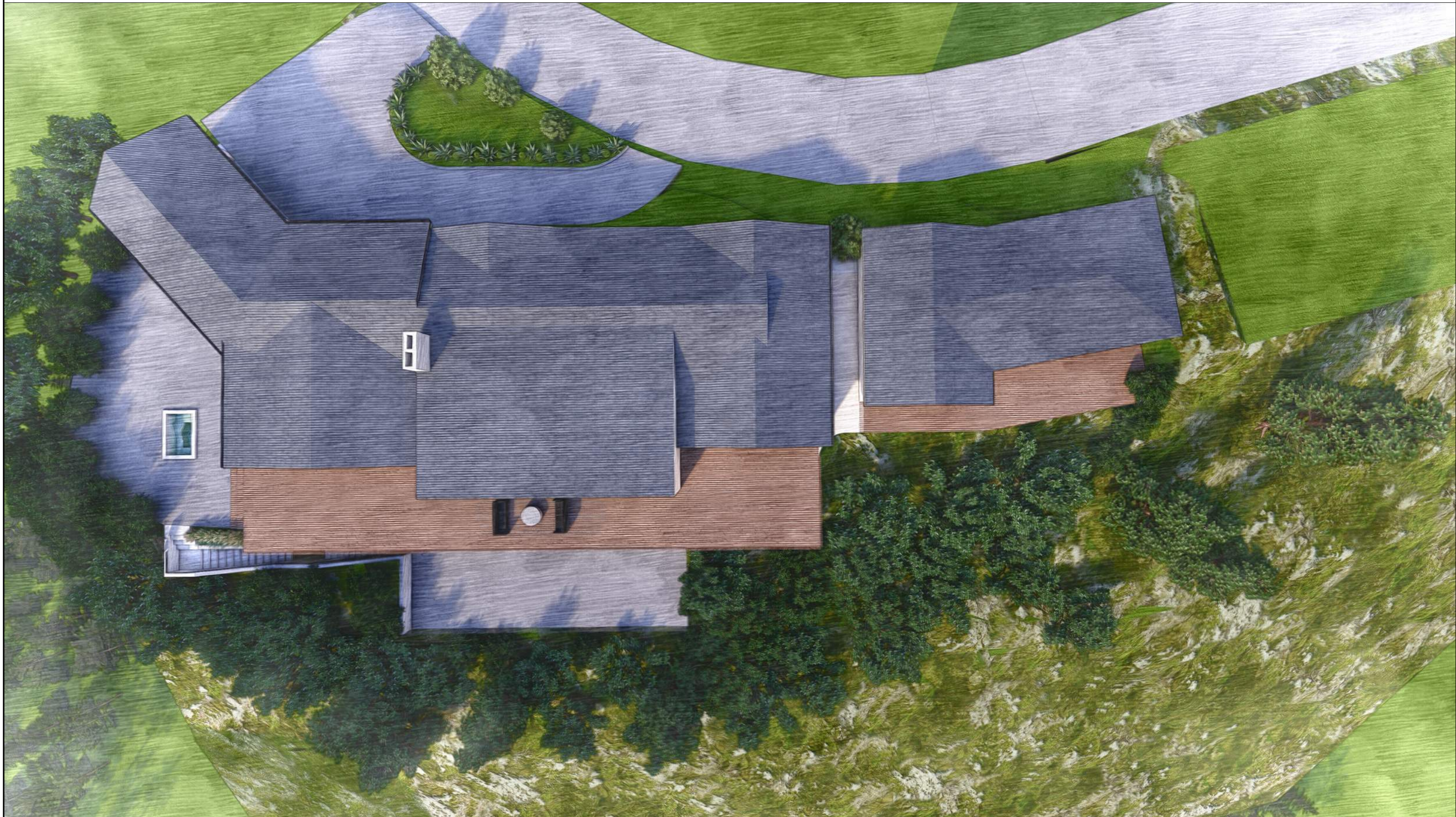
5 ROOF VIEW (N)
